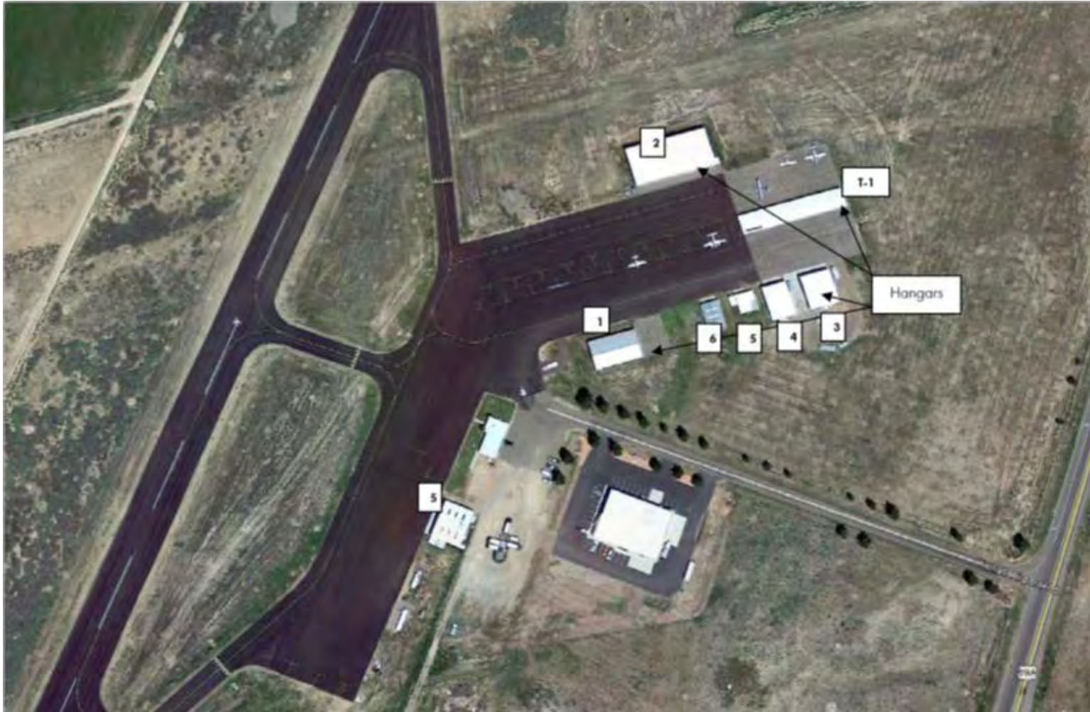
FIGURE 2-6 – KNB AIRPORT HANGARS
