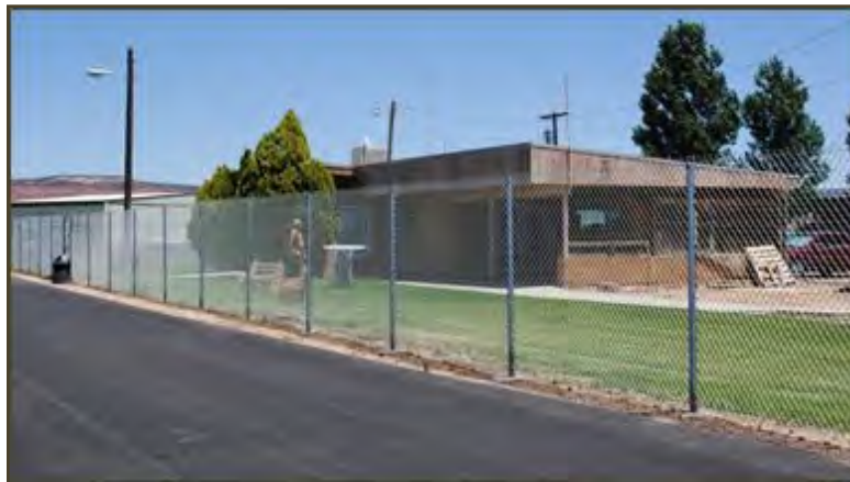
FIGURE 2-9 – EXISTING KNB TERMINAL BUILDING
